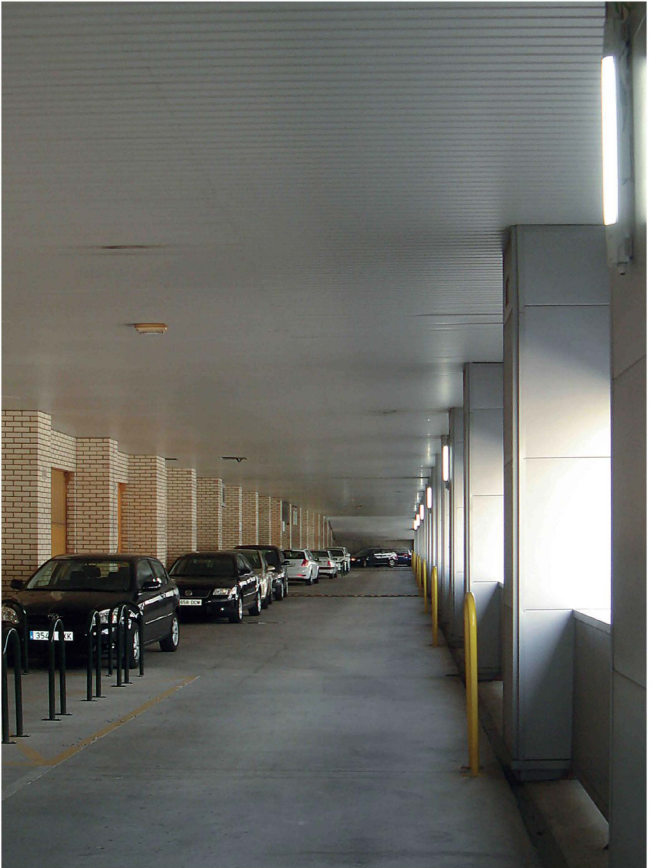
Ahorra Energia, Madrid (Spain)
